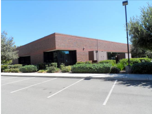
1. View southeast of Building 1445 west façade (north portion).
