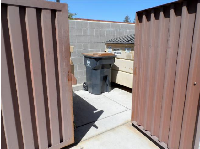
17. View of solid and recyclable waste bins in enclosure (typical).
