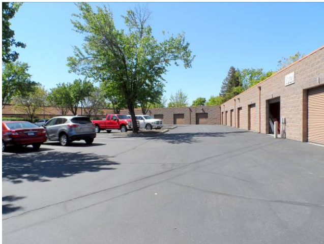
9. View west along Building 1921 southeast façade.
