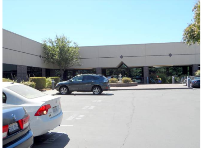
8. View southwest of Building 1850 northeast façade.
