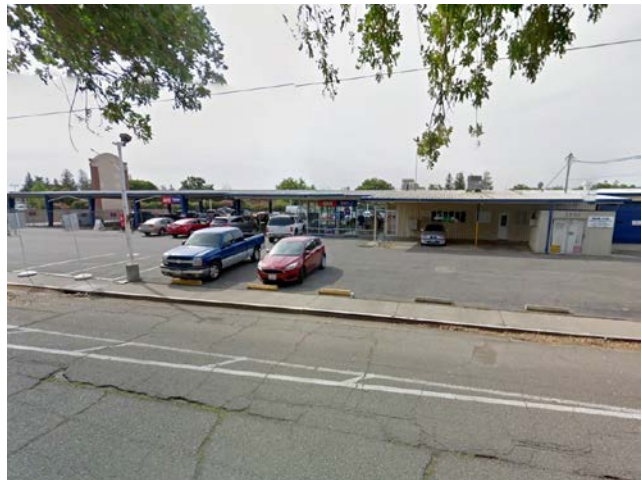
24. View of adjoining property to north across Interstate 80 freeway, Budget and Avis car rental businesses (closed LUST case site at 1800 Olive Drive).
