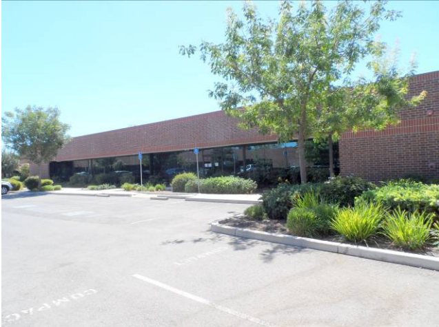
14. View south of Building 1940 northeast façade.
