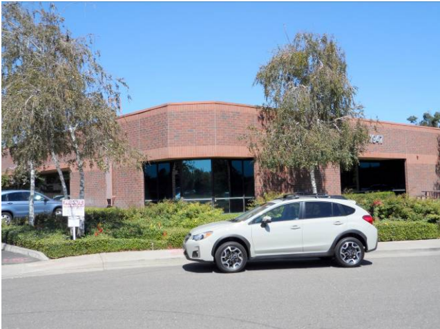
16. View northeast of Building 1947 south and west façades.
