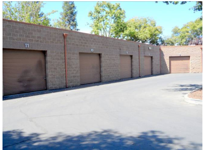
10. View west of Building 1921 east façade.
